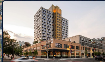
Newark Urby 2022 Build | 250 Units
