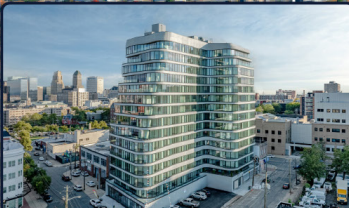
Hoyt Tower 2024 Build | 203 Units
