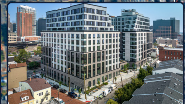
55 Union 2023 Build | 403 Units
