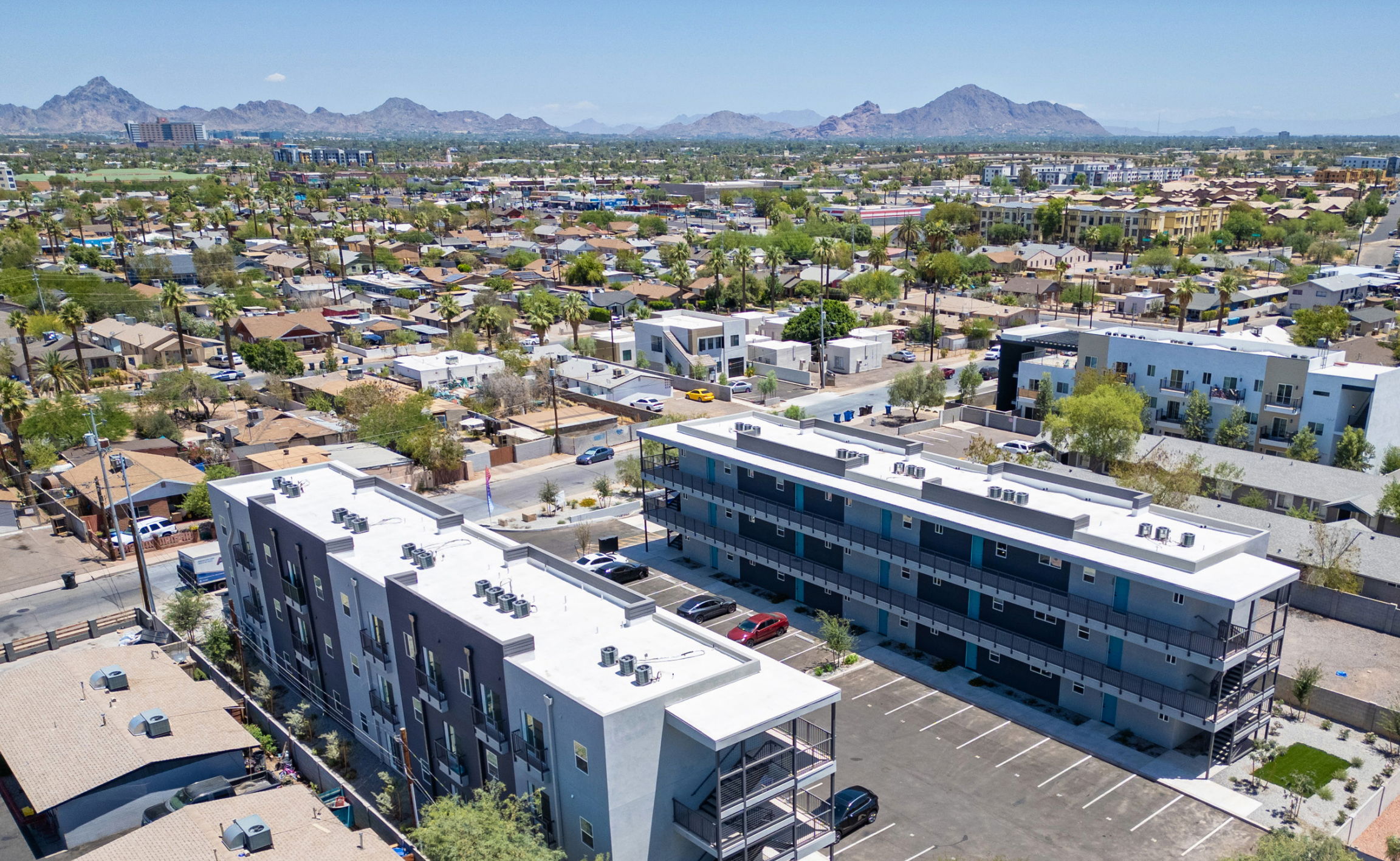
Newly Constructed Asset in Garfield District
