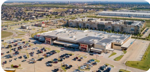
North: Neighboring a newly developed H-E-B, Texas's leading grocery chain.
