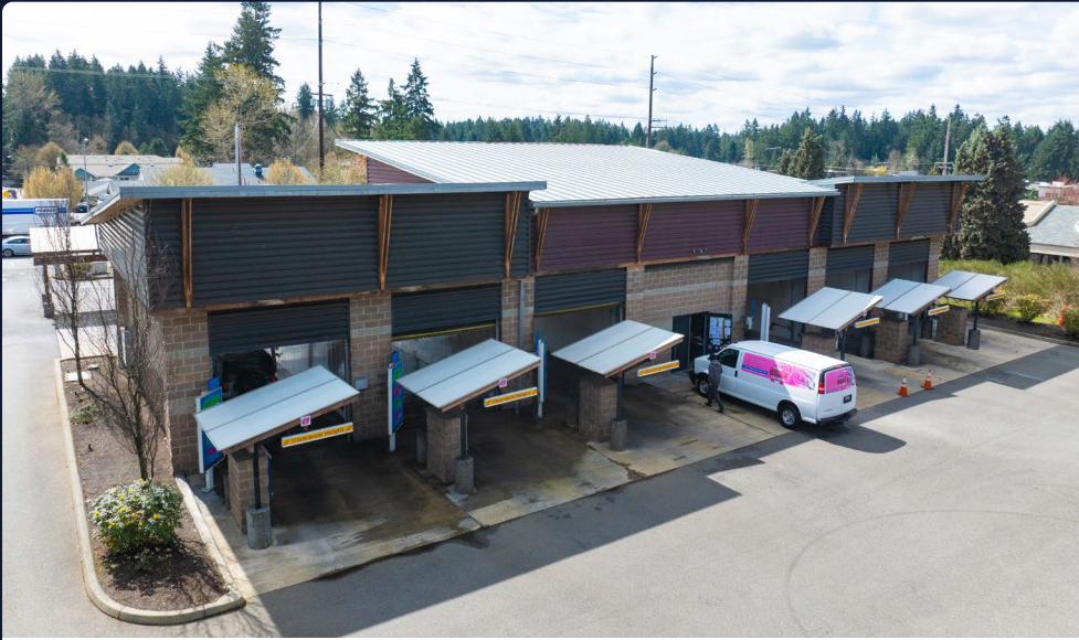
6 automatic wash bays
