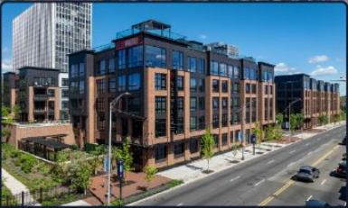
Vermella Broad Street 2024 Build | 296 Units
