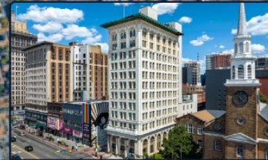
Indigo Residence 2023 Build | 106 Units
