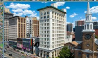
Indigo Residence 2023 Build | 106 Units
