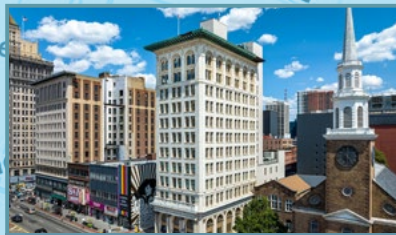
Indigo Residence 2023 Build | 106 Units
