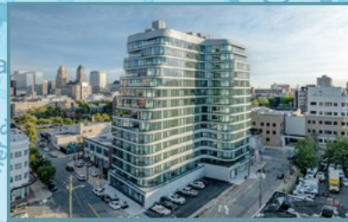
Hoyt Tower 2024 Build | 203 Units
