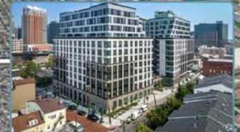
55 Union 2023 Build | 403 Units
