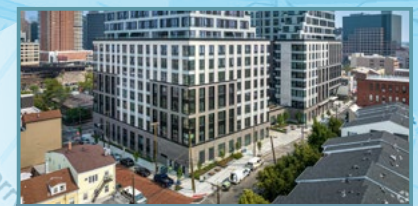
55 Union 2023 Build | 403 Units
