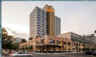
Newark Urby 2022 Build | 250 Units
