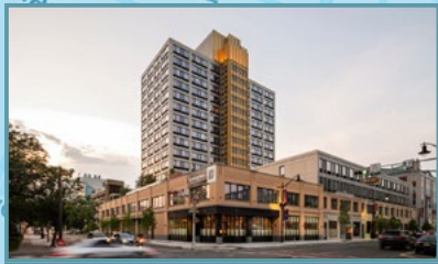
Newark Urby 2022 Build | 250 Units
