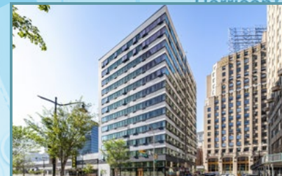
The Mercer 2025 Build | 110 Units
