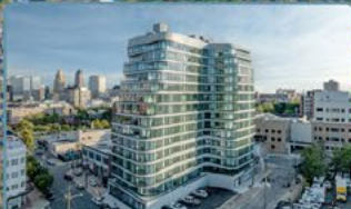
Hoyt Tower 2024 Build | 203 Units
