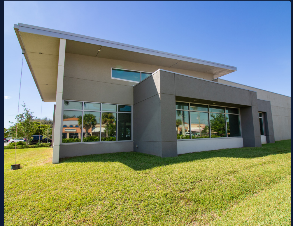
Exterior reflects stable, long-term tenancy appeal
