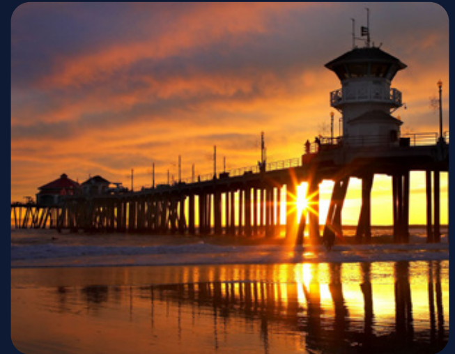
Huntington Beach Pier (HUNTINGTON BEACH)
