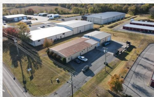
718 AIRPORT RD GALLATIN, TN
