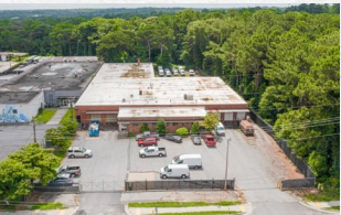
KROGER SERVICE FACILITY EAST POINT, GA
